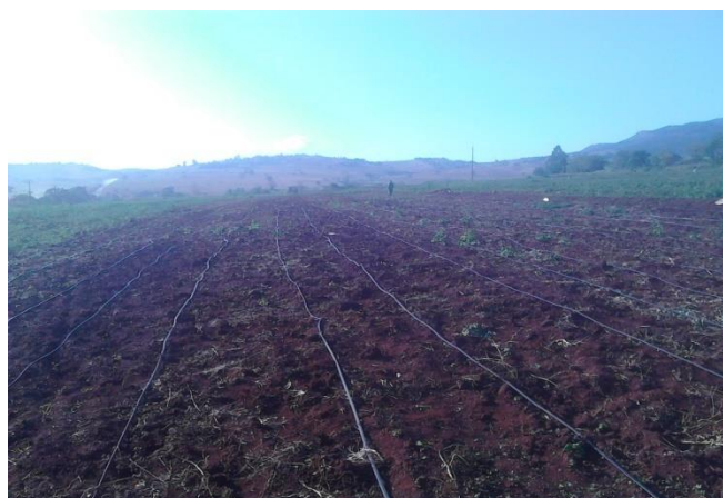
Plate 1. Drip irrigation installation (Mpatheni)
